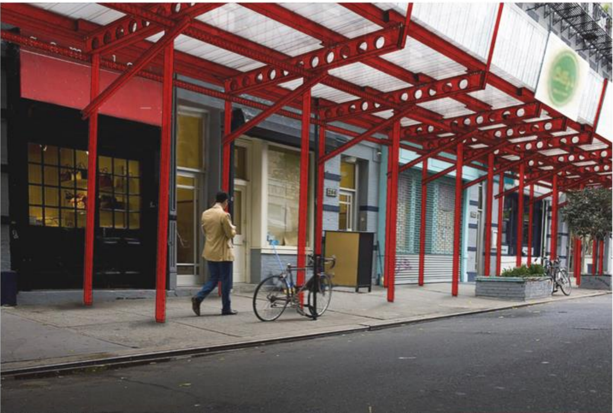
SCAFFOLDWING by Gannett Fleming Engineers and Architects, P.C. The scaffold's wing stretches out across the sidewalk, which directs sunlight to street level and drains rainwater. The roof is made of translucent polycarbonate panels which are light and airy. Image: Gannett Fleming Engineers and Architects, P.C.
